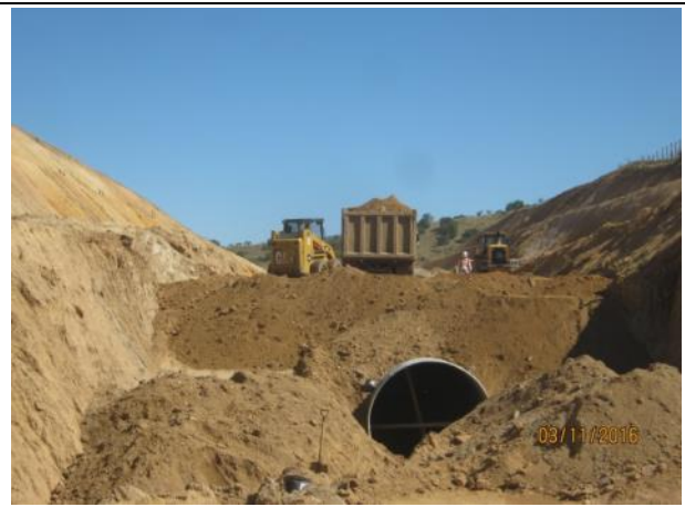
Relleno estructural, (Km 20,850 – Km. 21,100).
