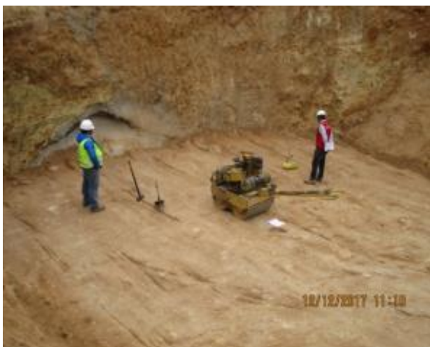
Relleno estructural, Km 7,060.
