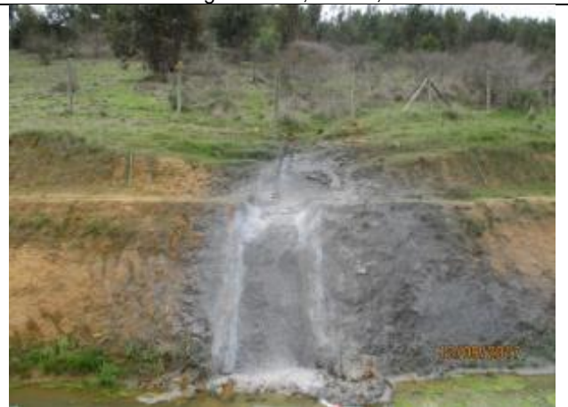
Descarga a canal, Km 23,820.
