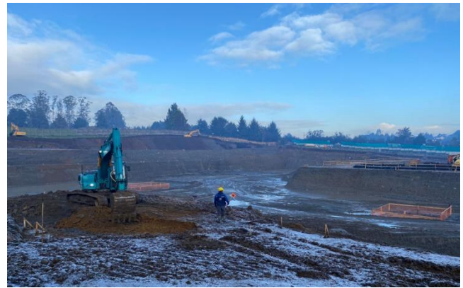
Hospital Puerto Varas
