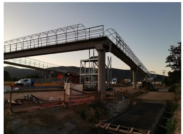
Pasarela Peatonal San Vicente, DM 76.800
