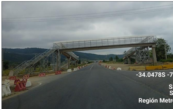
Dm 76.760 Pasarela Peatonal San Vicente
