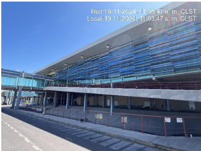
Vista Sector Air Side.
