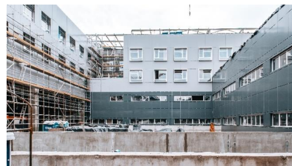
Fachada interior HDS
