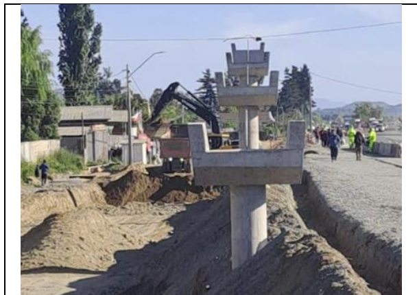
Pasarela peatonal Santa Inés, Dm 70.700
