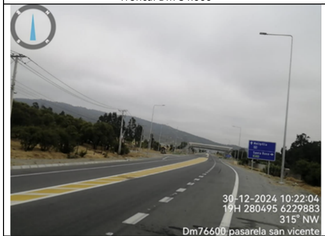
Pasarela Peatonal San Vicente, Dm 76.600
