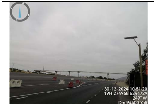
Pasarela Peatonal Central Rapel
