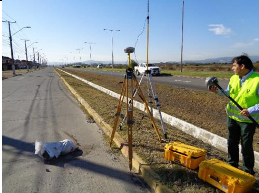
REPLANTEO PRs AUXILIARES Z-1, SECTOR A
