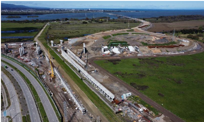
Vista General - Sector A
