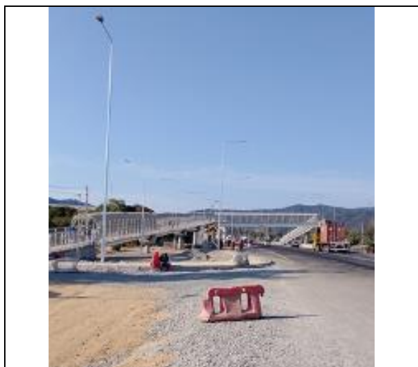
Pasarela Peatonal Santa Inés, Dm 70.700
