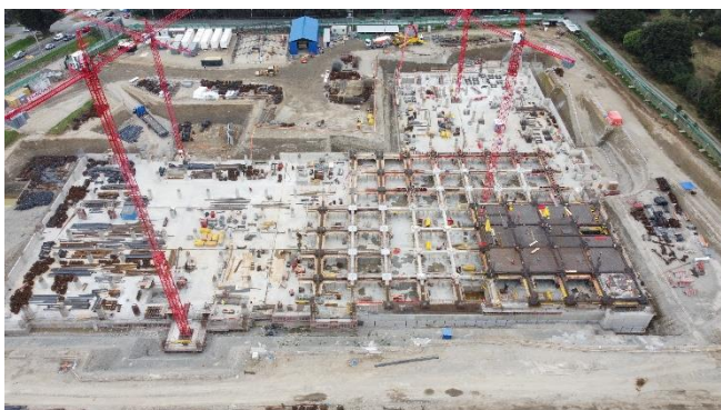
Hospital Puerto Varas
