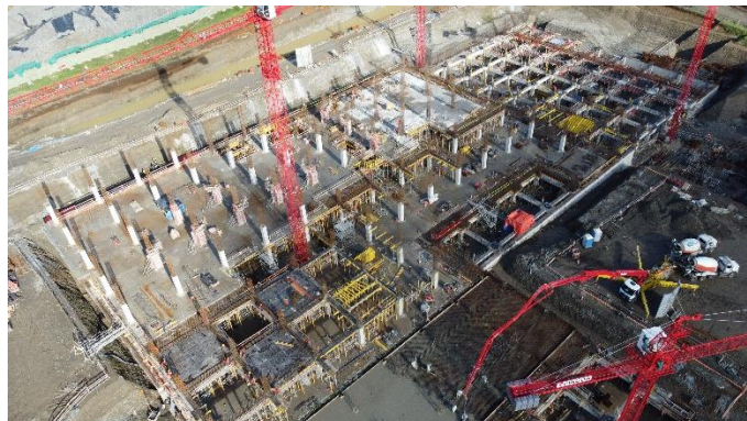
Hospital Puerto Varas
