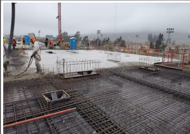
Hormigón Losa Cielo N3 (Sector E)
