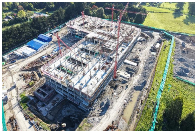
Hospital Puerto Varas
