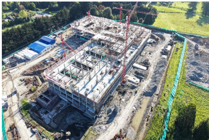
Hospital Puerto Varas
