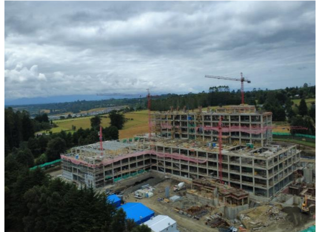
Hospital Puerto Varas
