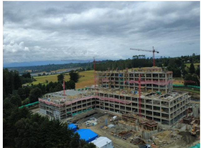
Hospital Puerto Varas
