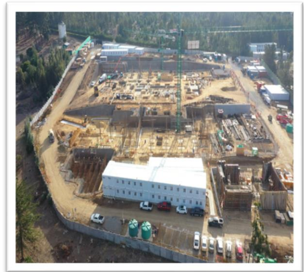
Vista General Faena Vista 1
