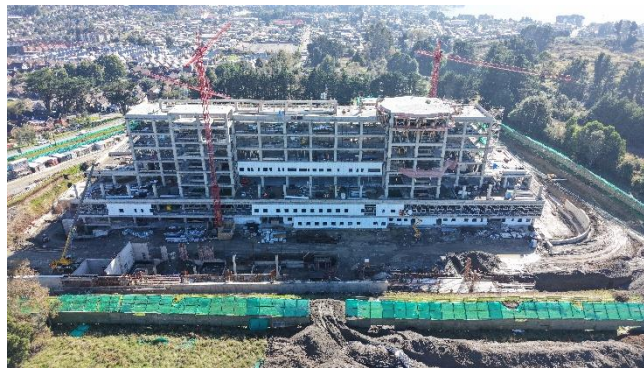
Hospital Puerto Varas
