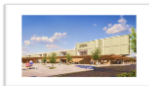
Hospital de Rengo
